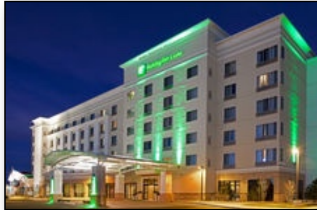
Holiday Inn at DIA 6900 Tower Road, Denver, CO
